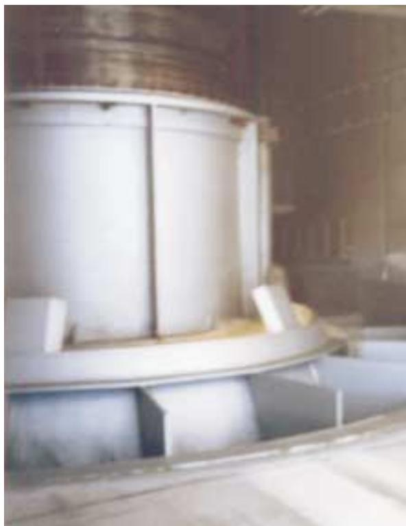
*A generator being placed on a turbine during project construction.*
