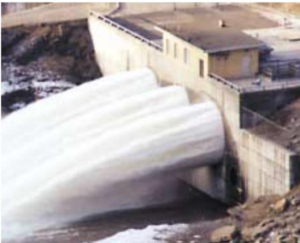
*The three tunnels shown here are set at the bottom of the dam allowing strong capacity for hydroelectric power generation.*
